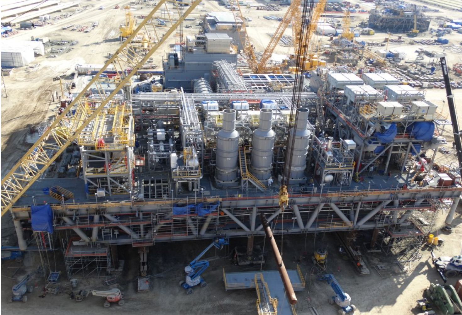
3 X CIRCULAR WHRUs on SOLAR TAURUS GT's FOR LLOG DELTA HOUSE PLATFORM, GoM, 2012
